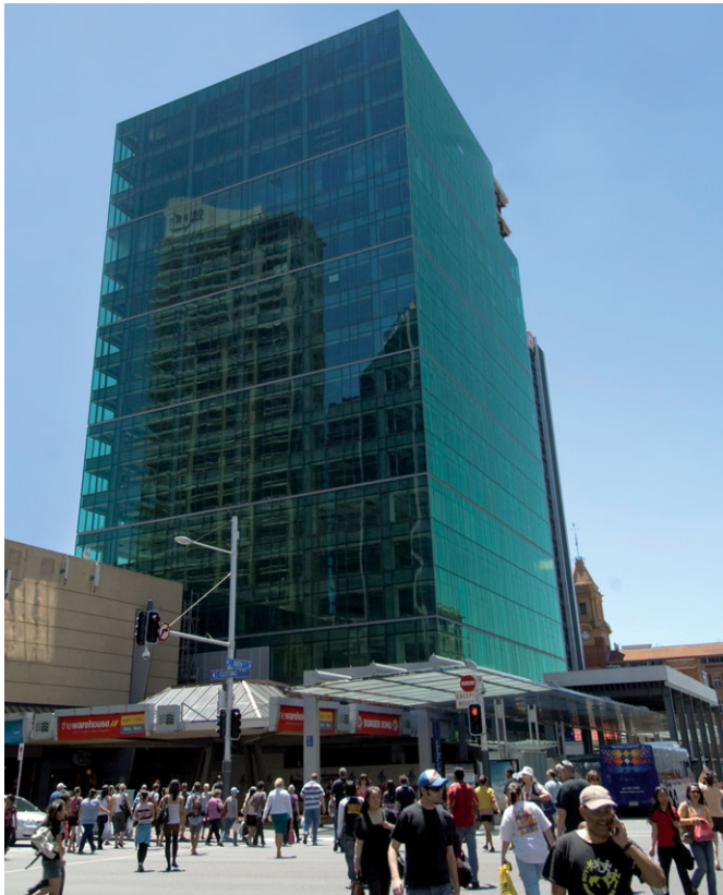
ComFlor employed in construction at Twenty-one Queen Street
