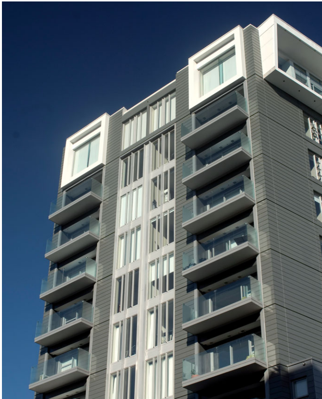
ComFlor employed in construction of Wellington's Bellagio Apartments
