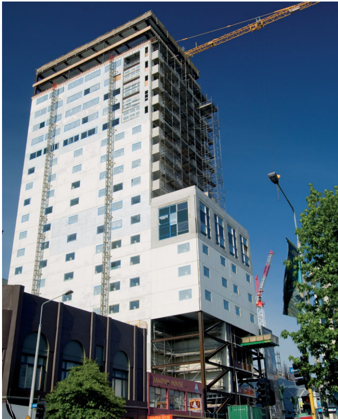
ComFlor makes for quick construction on C1 Towers
