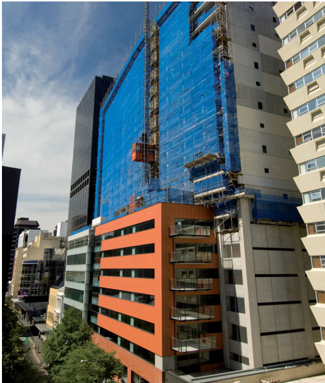
ComFlor allows quick simple construction on the Chews Lane project.
